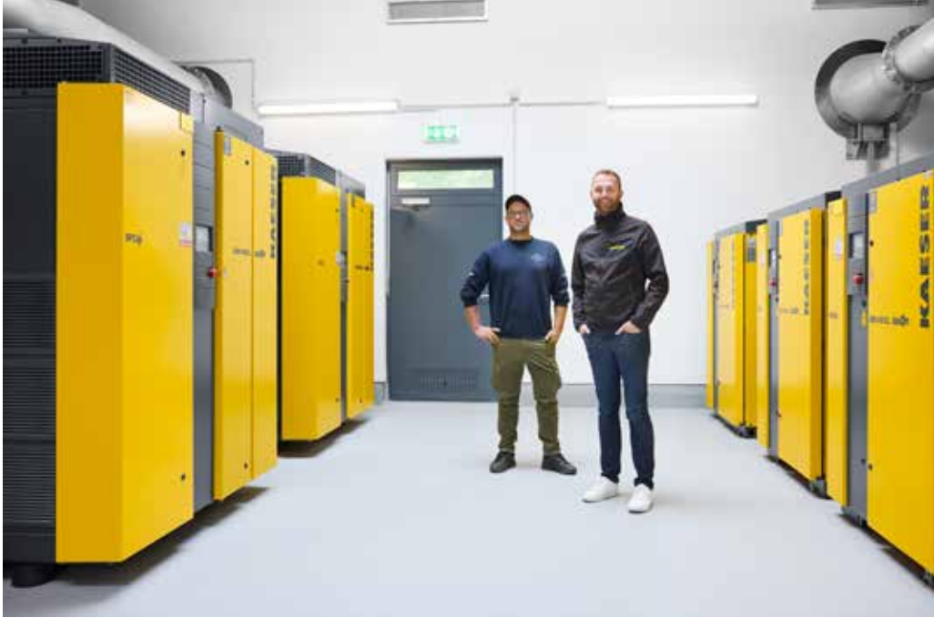
Image above: The SIGMA AIR MANAGER 4.0 operates in perfect coordination with the process control system. Image right: Five variable-speed KAESER rotary screw blowers supply air to the activated sludge tanks. To front: Florian Utz (Operations Manager, Forchheim wastewater treatment plant) and Matthias Sienerth (Sales Engineer, KAESER).
