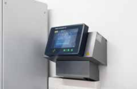
Image above: The SIGMA AIR MANAGER 4.0 operates in perfect coordination with the process control system. Image right: Five variable-speed KAESER rotary screw blowers supply air to the activated sludge tanks. To front: Florian Utz (Operations Manager, Forchheim wastewater treatment plant) and Matthias Sienerth (Sales Engineer, KAESER).
