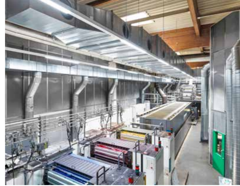
Compressed air is one of the most important energy sources for running modern printing and finishing equipment.
