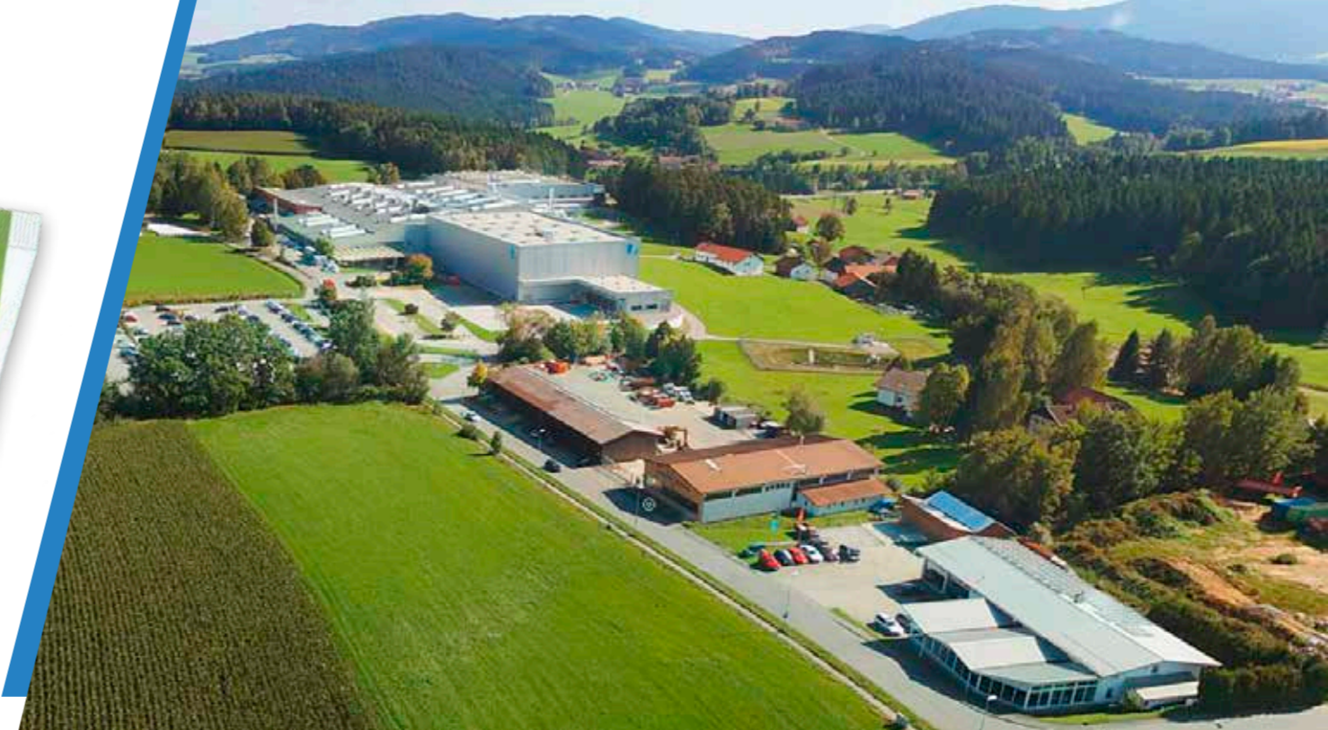
The LINHARDT facility in Viechtach, Lower Bavaria, nestles amid a beautiful, verdant landscape.
