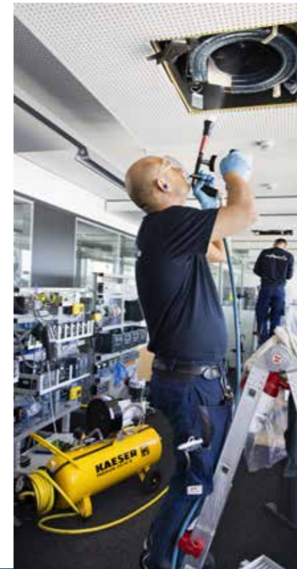
Left: The 'Eisschmitt Truck' transports the MOBILAIR compressor and all necessary dry ice blasting equipment. Right: On site at KAESER's Coburg facility – ventilation duct cleaning in action.
