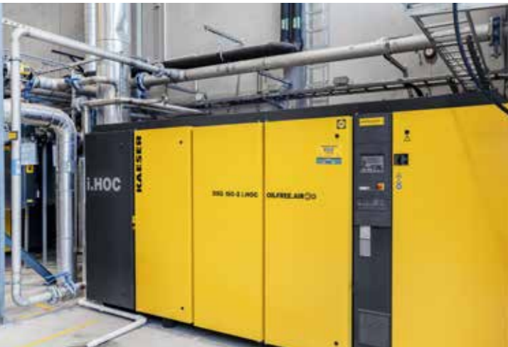
Bottom left: In total, there are three two-stage oil-free screw compressors DSG 180-2 with integrated i.HOC dryers. Bottom right: The SIGMA AIR MANAGER 4.0 is one of the reasons why Ringnes chose a compressed air station from KAESER.
