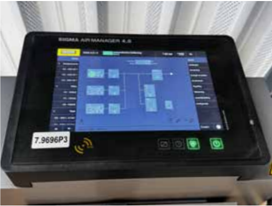
The SIGMA AIR MANAGER 4.0 ensures efficient operation and balances the workload between the machines evenly.
