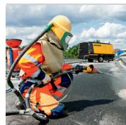
Many surface preparation and cleaning applications rely on compressed air, such as sand and dry ice blasting. In these cases, quality of the compressed air and its longevity, these specific applications require a constant supply of cool, condensate-free and technically oil-free compressed air that consistently meets the compressed air pressure and airflow requirements.
