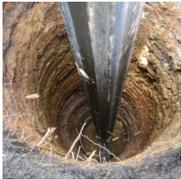
Pre-construction of major structures typically start with geotechnical drilling to assess the strata. Compressed air is required to transport the cuttings to the surface in a process which is referred to as flushing. When a DTH (Down-The-Hole) drill is being used, compressed air will also often be required to operate the drill.
