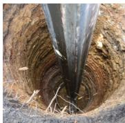
Pre-construction of major structures typically start with geotechnical drilling to assess the strata. Compressed air is required to transfer the cuttings to the surface in a process which is referred to as flushing. When a DTH (Down-The-Hole) drill is being used, compressed air will further be required to operate the drill.
