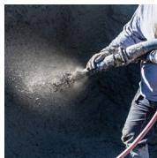
Compressed air is pivotal in achieving good concrete compaction in shotcreting and concrete vibration. For optimum results, the compressed air supply must reliably meet the pressure and airflow requirements, delivering cool and condensate-free compressed air. Shotcreting additionally requires technically oil-free compressed air that consistently meets the compressed air pressure and airflow requirements.
