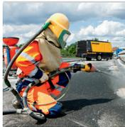
Many surface preparation and cleaning applications rely on compressed air, such as sand- and dry ice-blasting. For maximum productivity and equipment longevity, these specific applications require a constant supply of cool, condensate-free and technically oil-free compressed air that consistently meets the compressed air pressure and airflow requirements.
