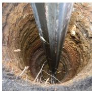
Pre-construction of major structures typically start with geotechnical drilling to assess the strata. Compressed air is required to transfer the cuttings to the surface in a process which is referred to as flushing. When a DTH (Down-The-Hole) drill is being used, compressed air will further impact pneumatic tool productivity and service life.
