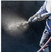
Compressed air is pivotal in achieving good concrete compaction in shotcreting and concrete vibration. For optimum results, the compressed air supply must reliably meet the pressure and airflow required, delivered cool and condensate-free compressed air. Shotcreting additionally requires technically oil-free air.
