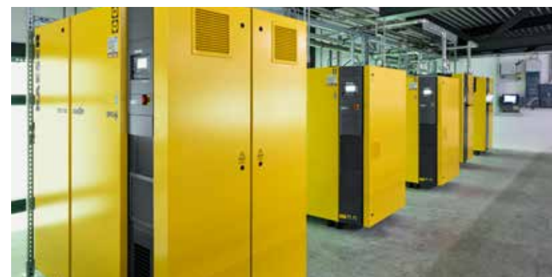
Top image: The in-house wood gasifier (Heizo E-Power) generates electricity and heat from wood chips on demand. Bottom image: The compressed air station is located on a mezzanine gallery overlooking the production area in the new hall.
