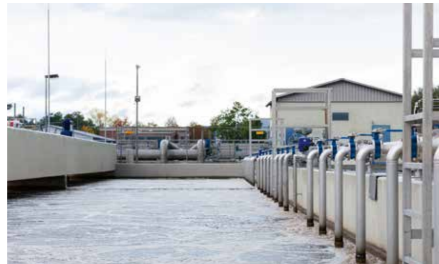
The refurbished aeration tanks.
