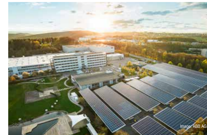
Image left: The new variable-speed CSDX 175 SFC rotary screw compressor meets the IES2 system efficiency level. Image right: The new photovoltaic system supplies around 1,100 MWh of carbon-neutral electricity per year.
